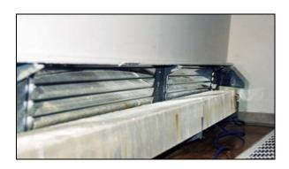
Using the same procedure, take the next sized section and fit it to the wall making sure that the edges line up to the Heat Reflector already installed.
