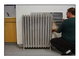
Peel the cover from the tape. Take one Heat Reflector and gently slide it behind the heating unit, being careful not to touch the wall. Once you have the Heat Reflector lined up and level, take the installation cane and gently press down on the vertical tracks (starting at the top) until the Heat Reflector is firmly fixed to the wall. It is best to work from the middle outward. Do not press too hard or you may puncture or flatten the ridges.
