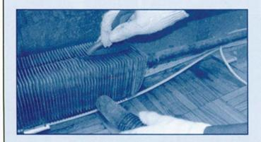
"We've found that a three-part approach works best for maximizing the heating efficiency of boiler systems", says Young. "In addition to an initial assessment of existing boiler and control equipment, followed by cleaning convectors, then installing reflectors, we also
